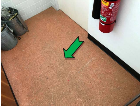
Photo 1. Interior, kitchen, beige floor coverings – non asbestos-containing sheet vinyl.
